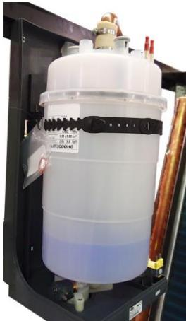
Modulating steam humidifier with immersed electrodes fitted with safety and running accessories. The accessory is factory installed and requires only water filling connection.
