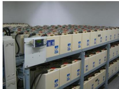
BLMG installation with a total of 540 batteries (6 V 150 Ah)
